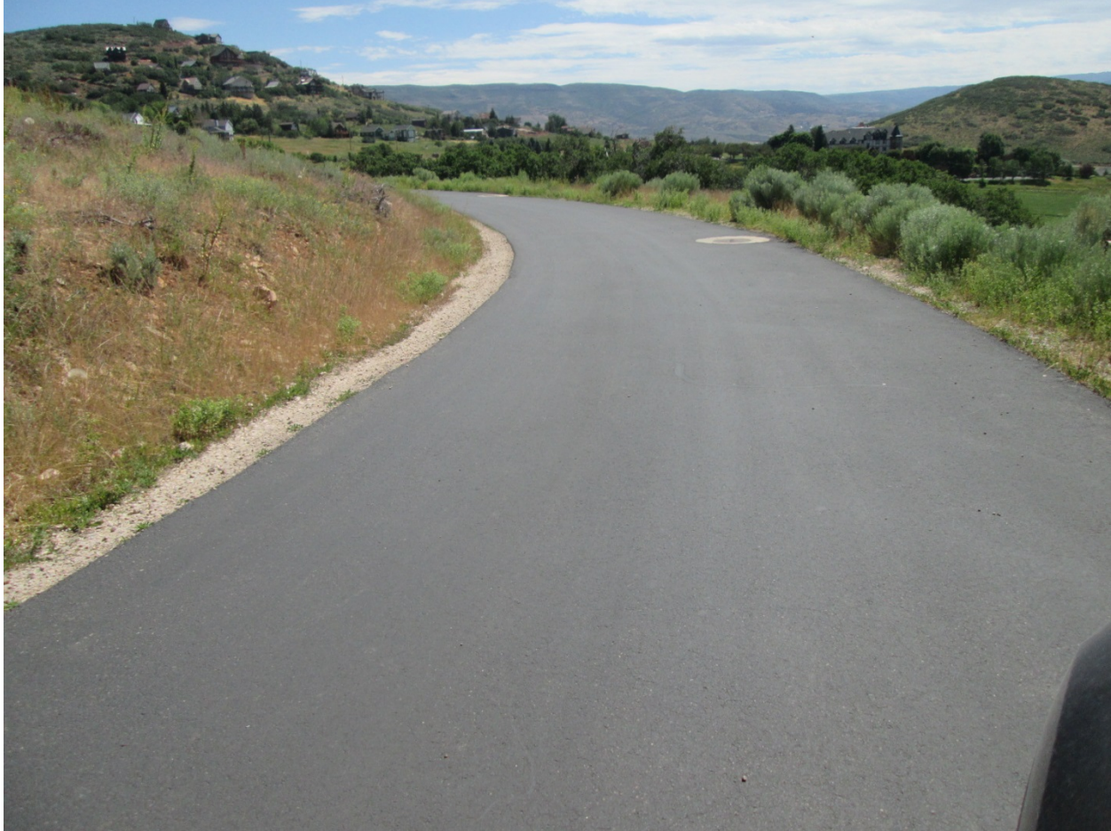
Photo 3. Very Good Condition – Luzern Rd from Luzern Rd to Luzern Rd (RSL = 14 years)
