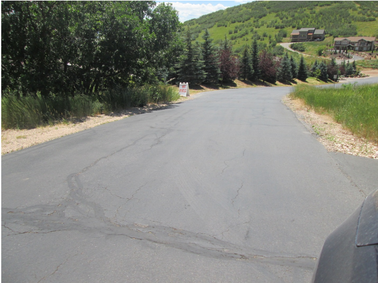
Photo 1. Fair Condition – Interlaken Dr from Interlaken Dr to Edelweiss Ln (RSL = 8 years)
